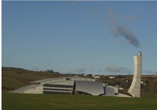
Isle of Man (for reference, the stack is 70m high)
